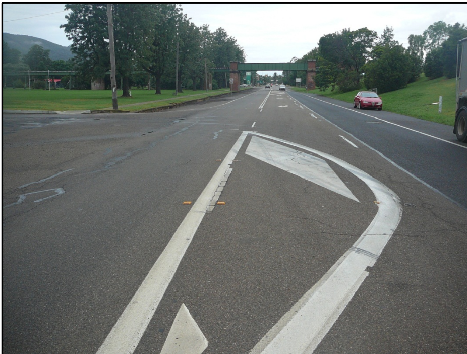
■ Photo 4 Photo shows the sheltered right turn lane on Peel Street at O'Connell Street
